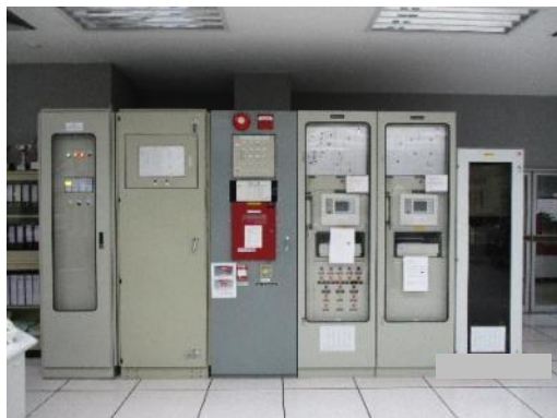
Master Fire Alarm Control Panel
