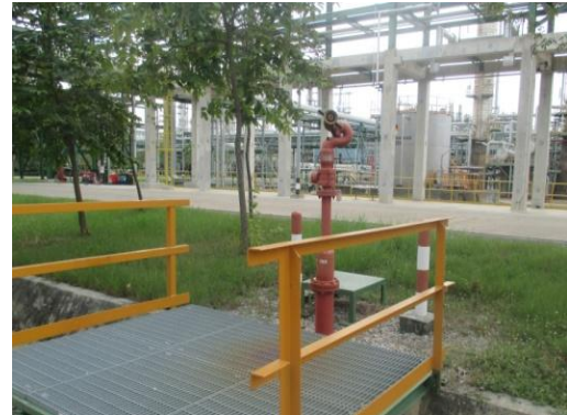
Water Hydrant with Monitor
