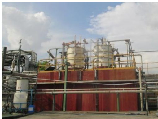
Neutralization Tank
