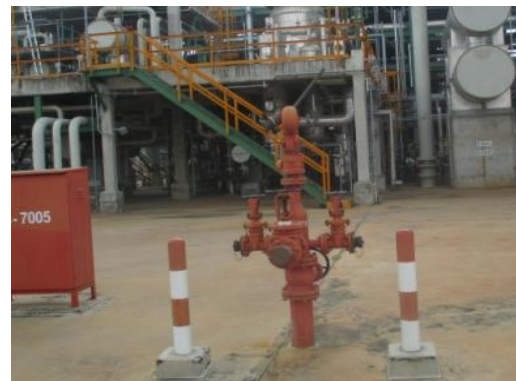
Water Monitor with Remote
