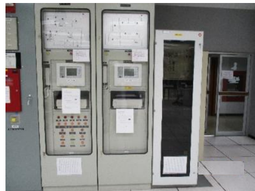
Slave Fire Alarm Panel
